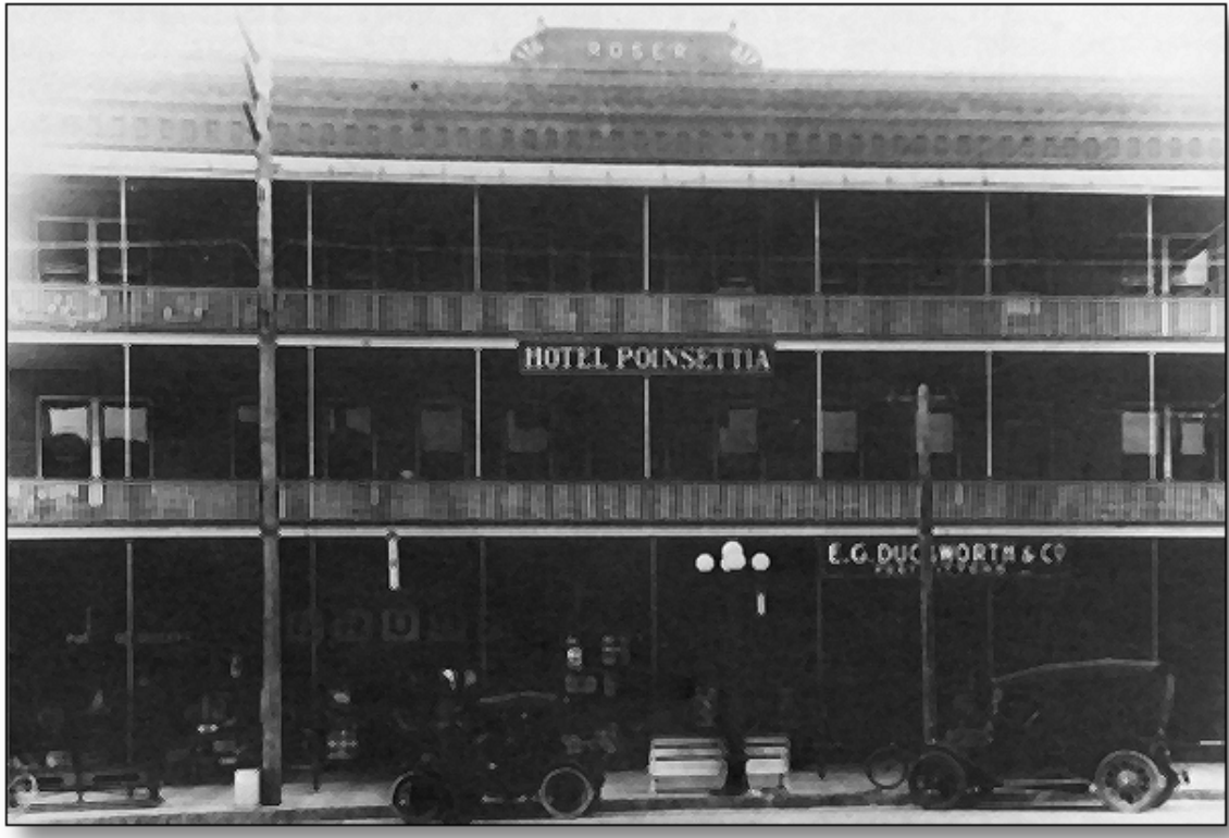
The Hotel Poinsettia on Central Avenue, 1914.
